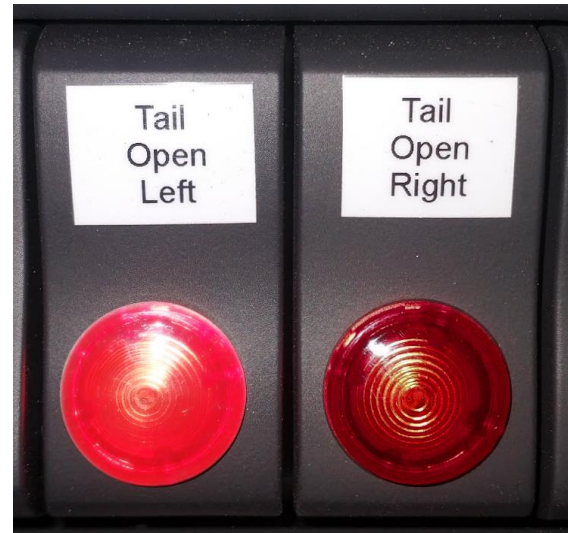
Fig 2. Check if warning light illuminates
